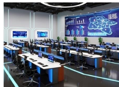
Control Room Furniture Solution
